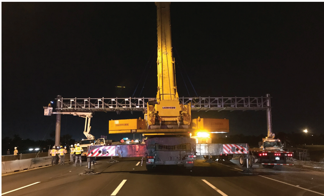
Overhead sign structure installation
