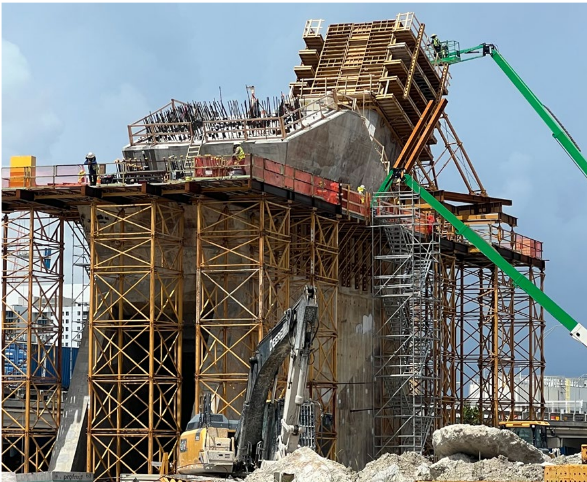
Ongoing work at the signature bridge center pier structure
