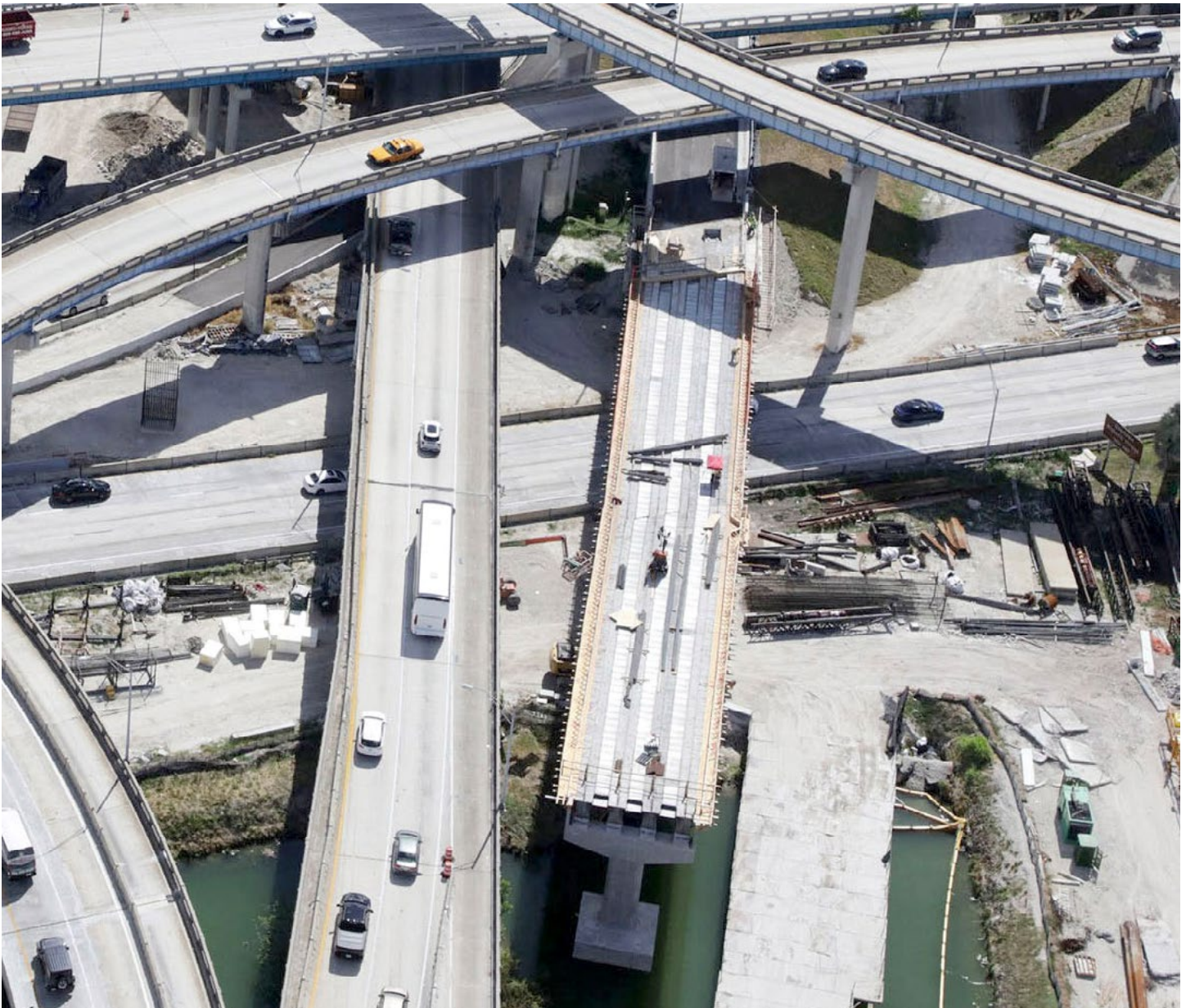
Eastbound SR 836 connector bridge to I-395 ready for concrete deck pour
