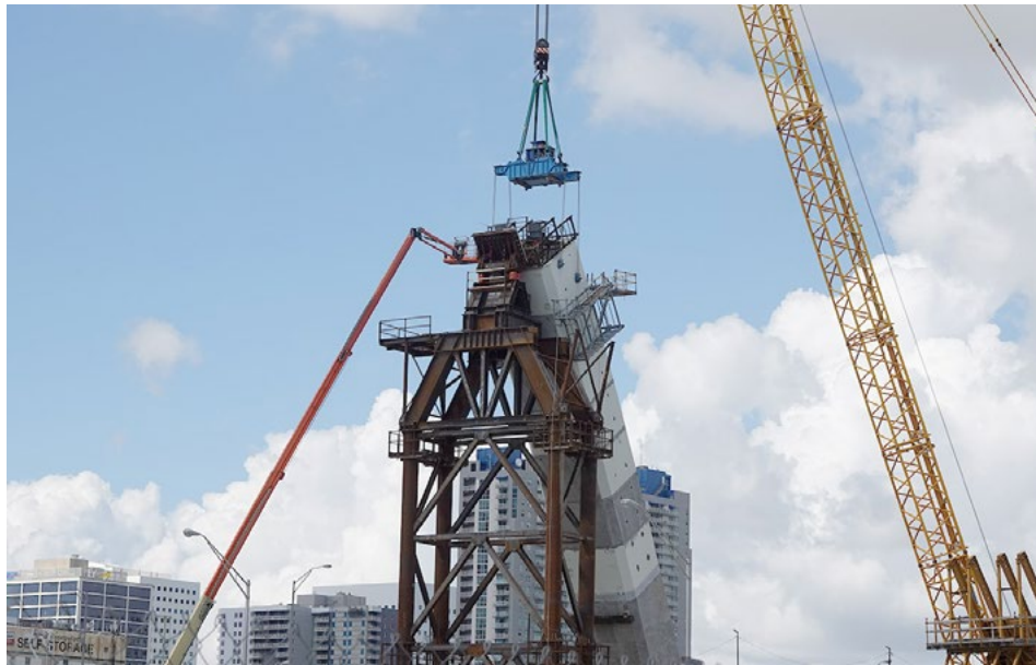
Installation of a precast arch segment for the I-395 signature bridge
