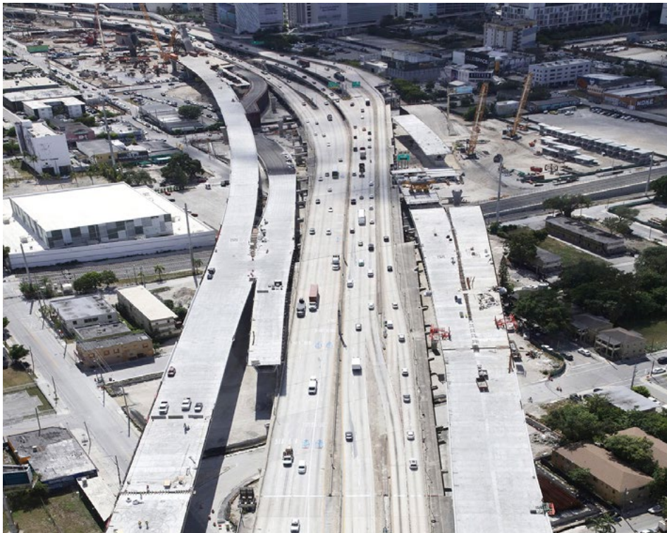
Ongoing construction of new I-395 segmental bridges
