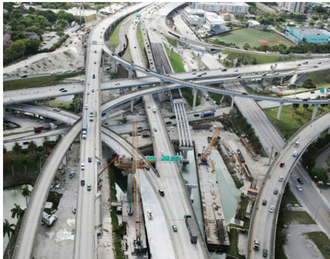
Ongoing bridge and roadway construction at the SR 836/I-95/I-395 Interchange core.
