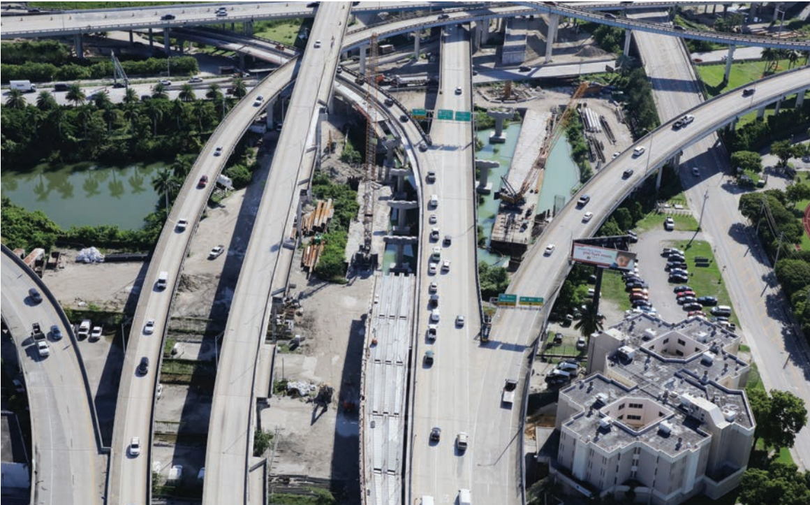
Widening of the eastbound SR 836 ramp to northbound I-95
